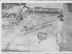
ON THIS spot above, Lago's cold storage building stood for thirty-one years. Slabs from ceiling and walls were lifted by a mobile crane and loaded on a low-boy. They may be dumped later on the harbor reef. E LUGAR aki tabata e sitio camina e edificio di Cold Storage tabata durante treinta y un aña. Planchan di plafon y mura y a worde lamá cu grua y cargá riba un "low-boy."
